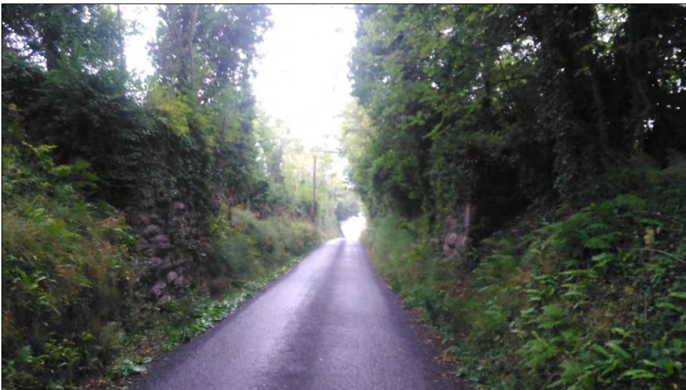
Plate 4: Remains of Railway Bridge S2-BH03
