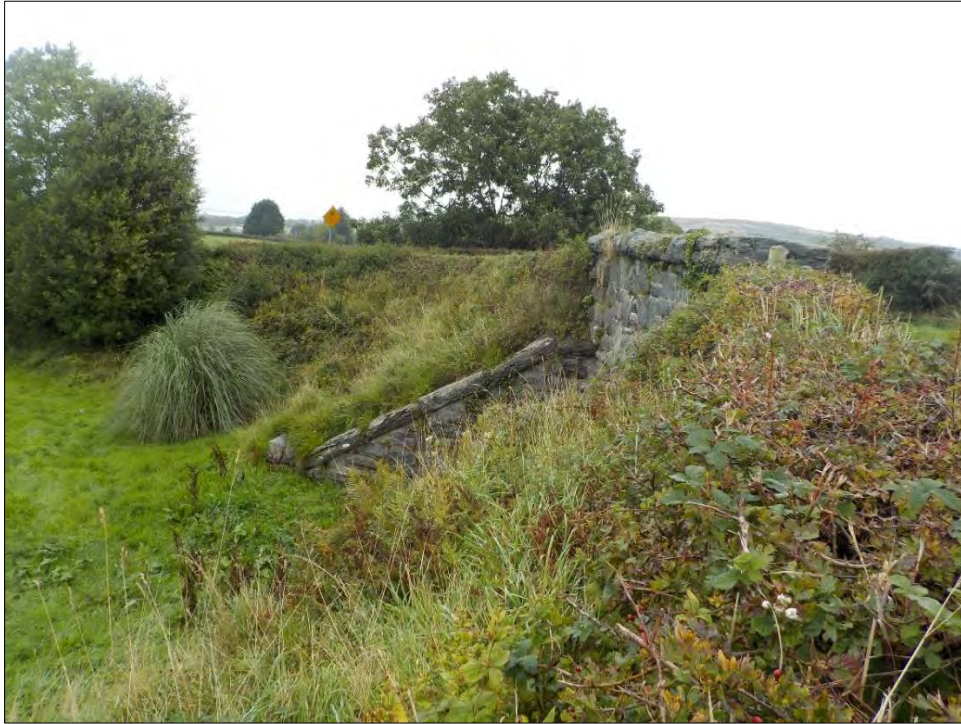
Plate 3: Pluck Railway (road) Bridge NIAH 40905337
